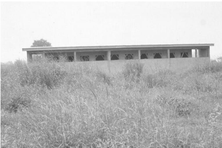
These new public latrines are too far from the market and have no cleaning system in place. Ease of maintenance and impact on the local environment are critical elements for proper planning of small-scale construction projects.
