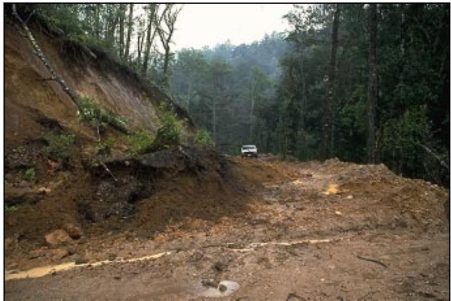
**Photo 1.3** A problematic road because of roadcut failures. Instability problems cause road user delays, and high maintenance or repair costs.
