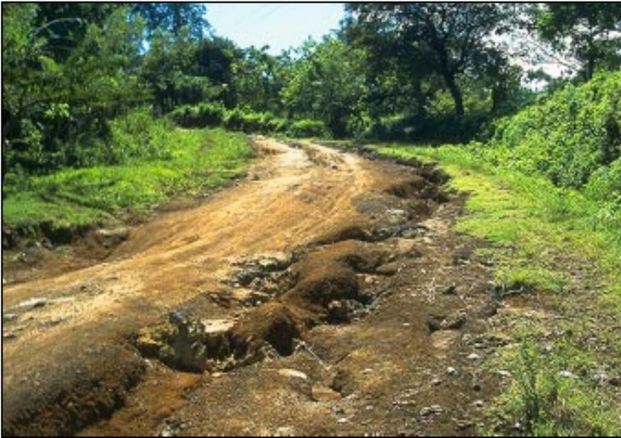
**Photo 1.2** A poorly drained road that has a rough driving surface for the users, it is a source of sediment, and it is relatively expensive to maintain.
