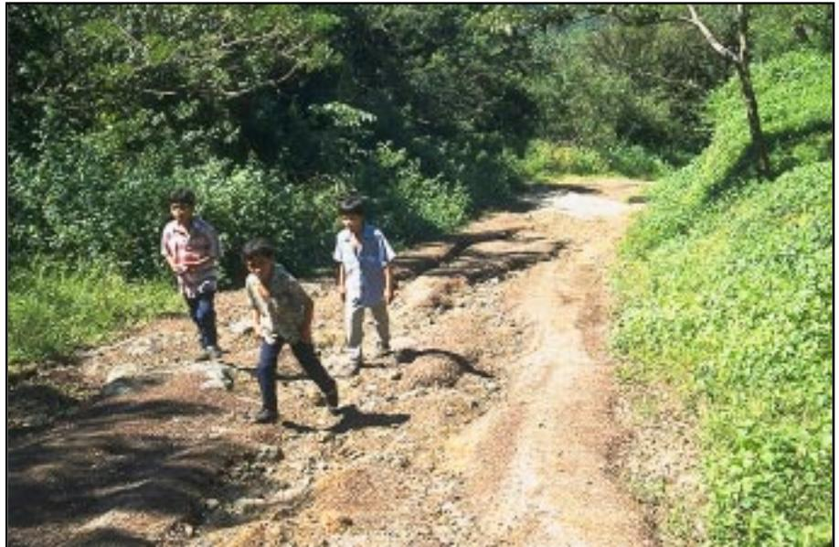
**Photo 2.4** Adverse environmental impact from road surface erosion caused by steep road grades and insufficient cross-drains. This road is also difficult to maintain.
