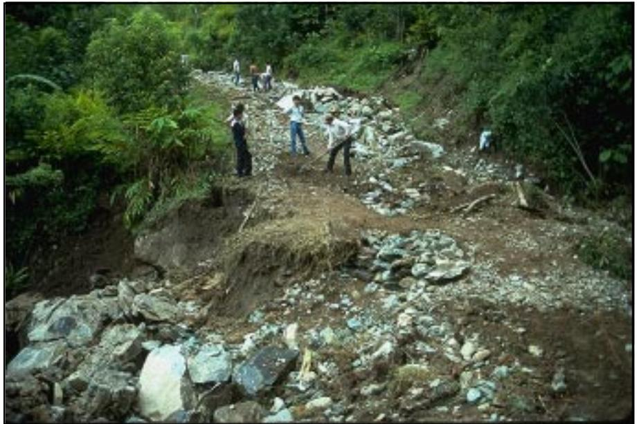
**Photo 3.4** A road that has been heavily damaged during a storm because of an undersized, plugged culvert pipe and no overflow protection.
