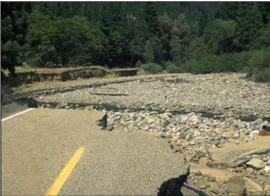
**Photo 3.3** A poorly located road, in the hazardous flood plain area of a river, that has washed out during a major storm event.
