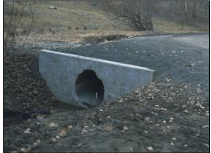
**Photo 4.6** A well designed and installed culvert with head walls for efficiency and fill protection.
