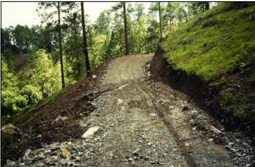
**Photo 4.3** Avoid constructing roads with steep grades or on steep side slopes. It is difficult to control drainage with steep road grades.
