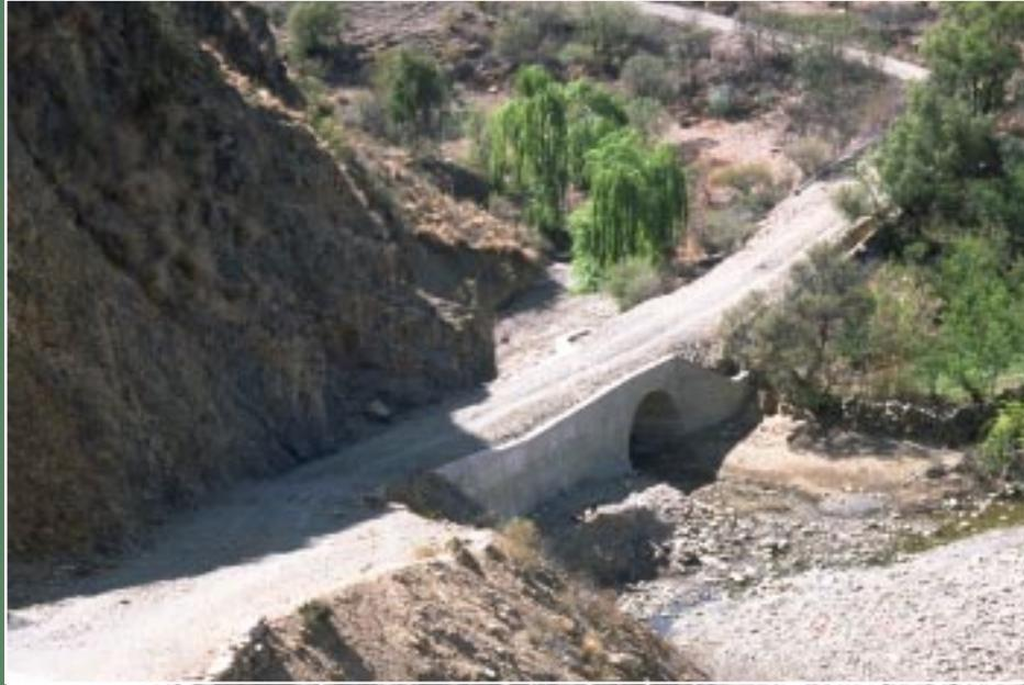
*A drainage crossing can be a critical and vulnerable point in the road if the drainage structure fails. Thus, drainage crossings must be designed to pass the appropriate storm flows plus debris or to survive overtopping.*
