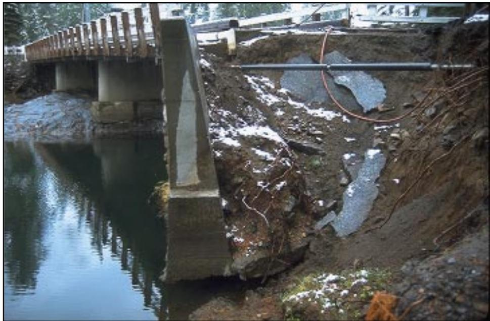
**Photo 6.1** Scour behind a bridge abutment caused by insufficient channel and stream bank protection during a flood.
