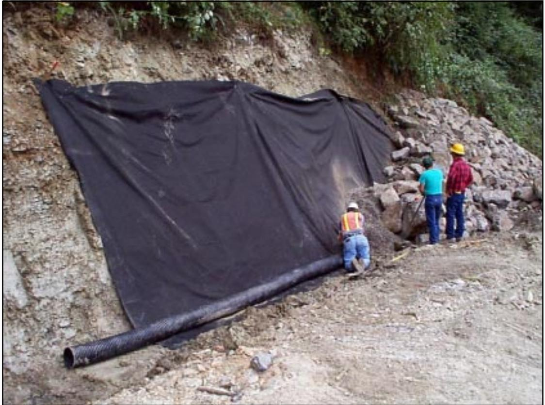
**Photo 6.5** A filter cloth (geotextile) backing behind a loose rock slope buttress to provide a filter for drainage and to prevent movement of fine soil into the rock. (Photo by Richard Van Dyke)
