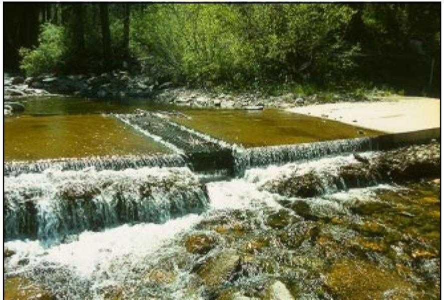
**Photo 9.5** Some fords can be designed as “low-water bridge” structures. They must be designed to be occasionally overtopped and have an erosion resistance deck and approaches. This structure is ideal for fish passage.
