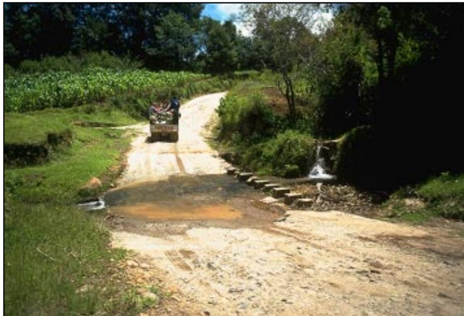
**Photo 9.1** Use armored low-water crossings, fords, or drifts as often as possible to cross low flows in broad, shallow natural drainages, thus avoiding the use of pipes. Note that part of this reinforced driving surface needs repair.
