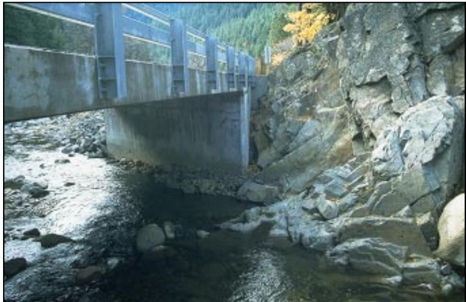
**Photo 10.6** Here is a well built treated timber bridge with good streambank protection and adequate span to minimize stream channel impacts. The freeboard is marginally adequate.
