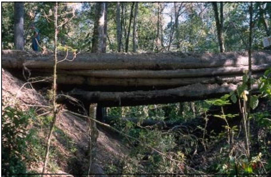
**Photo 10.2** A bridge structure typically offers the best channel protection by staying out of the creek. Use local material for bridges as available, considering design life, cost, and maintenance. Inspect bridges regularly, and replace them when they are no longer structurally adequate.
