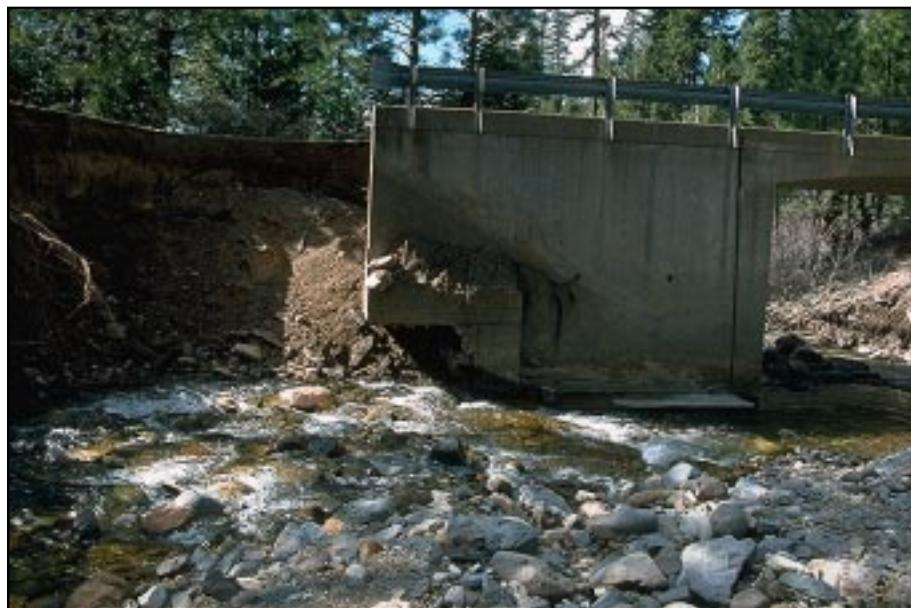
**Photo 10.3** Scour is one of the most common causes of bridge failure. Use an opening wide enough to minimize constriction of the natural channel. Locate the bridge foundation on bedrock when possible, or below the depth of scour, and use stream bank protection measures such as riprap.
