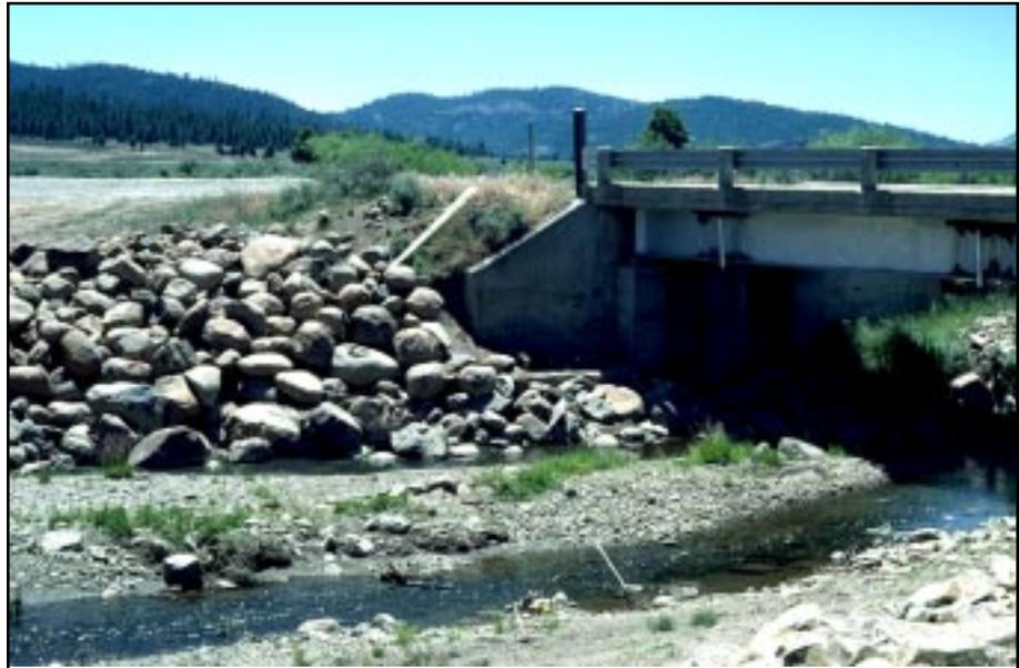
**Photo 10.5** Locate the bridge foundation on bedrock or on non-scour susceptible material when possible. When it is necessary to locate the bridge foundation on materials susceptible to scour, use a deep foundation or design the bridge with scour protection.
