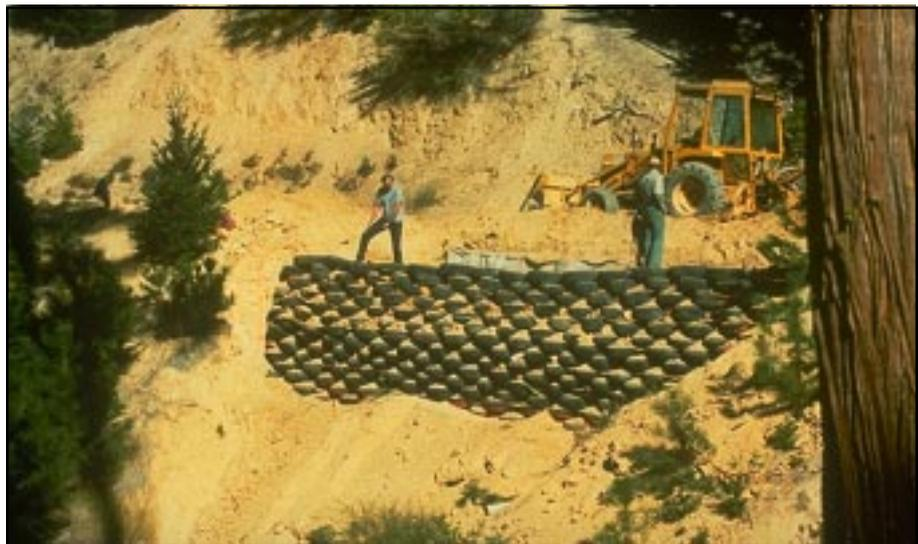
**Photo 11.12** A gabion retaining structure which will fail soon due to lack of a suitable foundation. All retaining structures, either mechanically stabilized earth (MSE) walls or gravity walls, require a **good foundation**.
