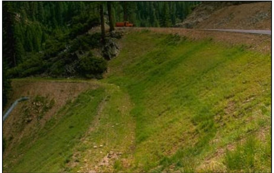
**Photo 11.5** Construct fill slopes with a 1 1/2:1 or flatter slope (to promote vegetation growth) and stabilize the fill slope surface. Use benches (terraces) on large fill slopes to intercept any flow of surface water.
