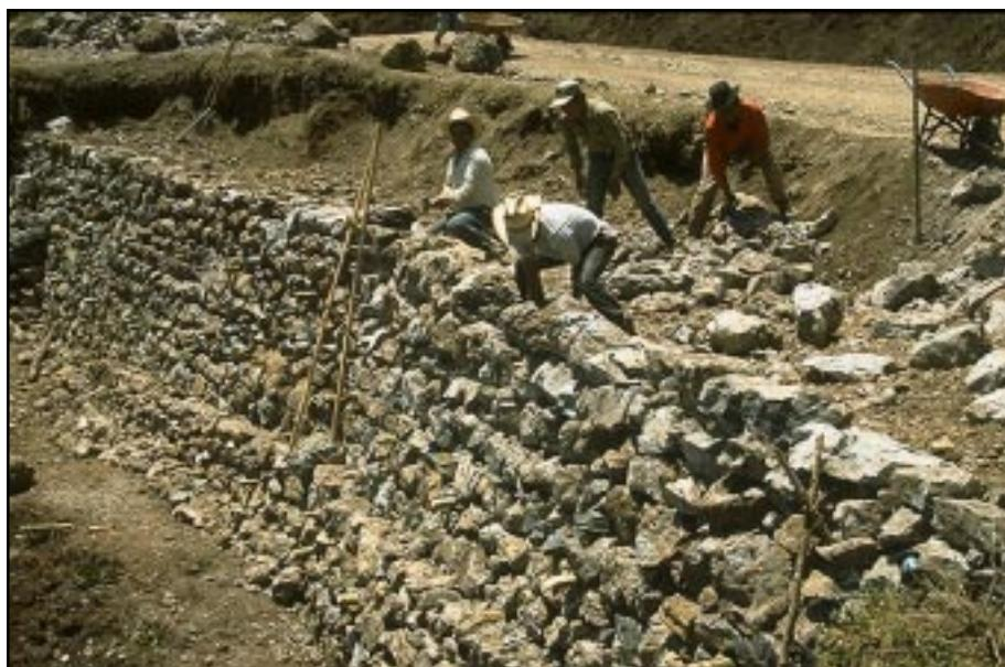
**Photo 11.8** Use physical slope stabilization methods, such as retaining walls, reinforced fills, or rock buttresses where necessary in areas of space limitation on steep slopes.
