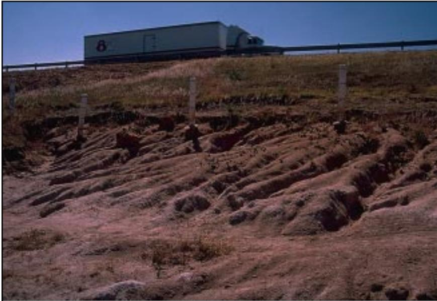
**Photo 13.2** Erosion on a slope adjacent to a highway due to lack of vegetation or poor land use practices. Note that vegetation is preventing erosion next to the highway.
