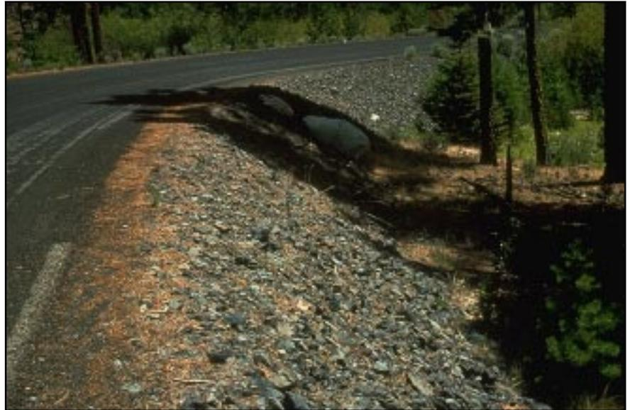
**Photo 13.8** Seed and mulch (cover for seed protection and moisture retention) applied to the ground surface to promote grass growth on barren areas, closed roads, and on erosive soils.
