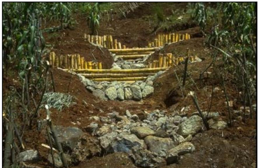
**Photo 14.4** Construct debris retention and gully control structures with a notched weir to keep flow over the middle of the structure, add scour protection at the outlet of each structure, and key the structures into the firm soil banks.
