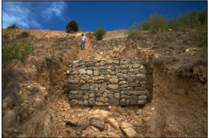
**Photo 14.3** An expensive but failed gabion gully control structure that was not properly keyed into the banks of the gully. Further, the flow was not kept over the protected middle of the structure.
